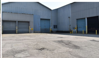
Drive-In & Dock Level Doors
